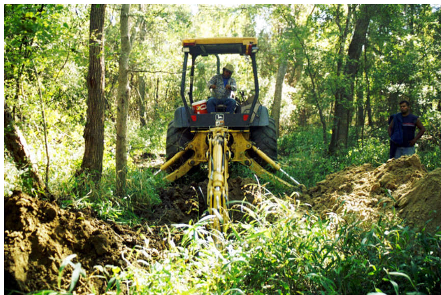
Figure 4-5. Armando Salinas conducted the trenching operations for the project.
