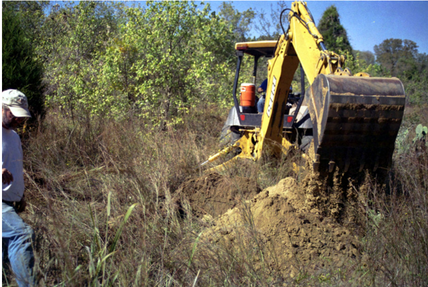
Figure 4-6. Monitoring backhoe trench excavations adjacent to Big Sandy Creek.
