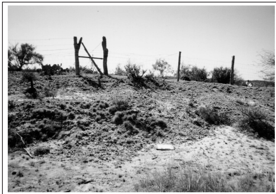
Figure 6. Photograph of eroded surface of site 41MV127.
