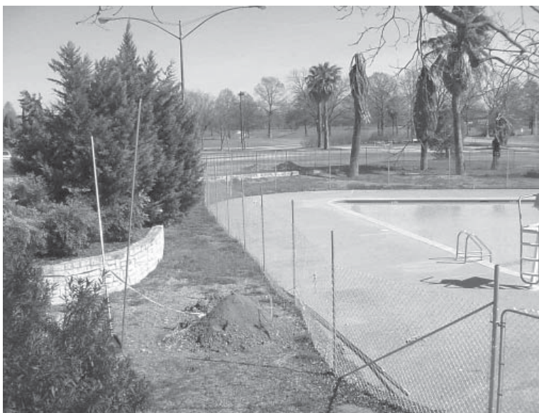
Figure 7-6. Unit 1 was placed near the west edge of the swimming pool; facing northeast.
