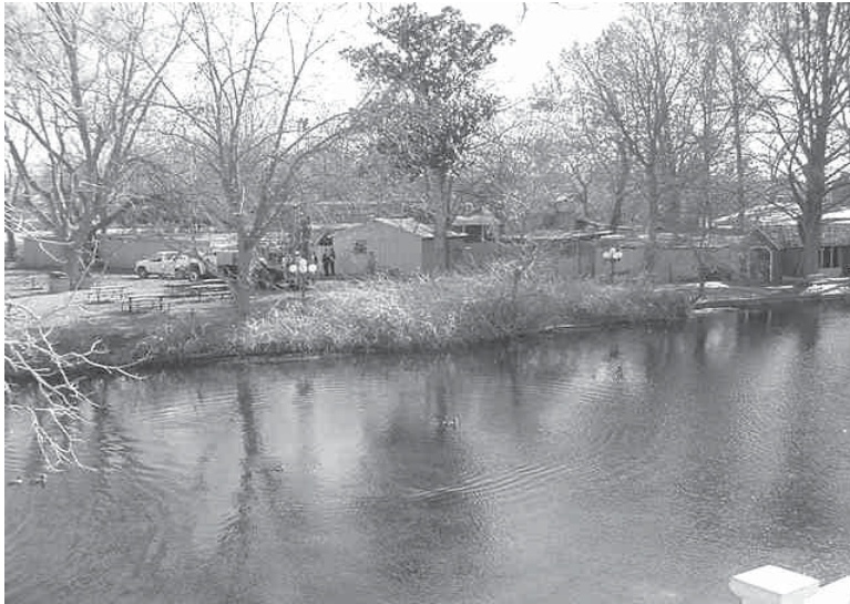
Figure 5-7. Core drilling in the pecan grove at Aquarena Springs.
