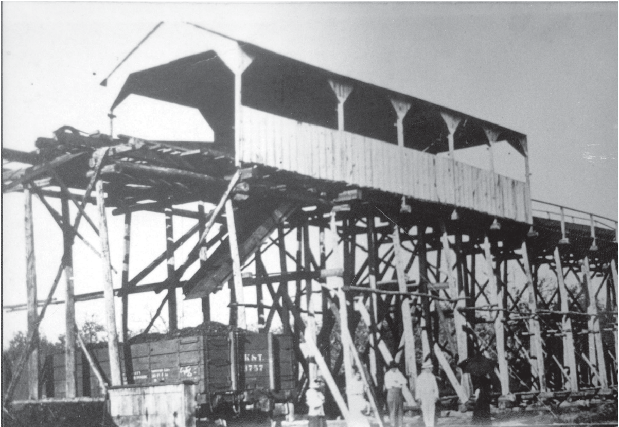
Figure 4-68. Graded tippel leading from slope mine in operation from 1914-1924. Lignite from the mine carts was dumped into MK&T railcars for transport to the main line 2½ miles southwest. (Photograph from the Camp Swift historical files, AGTX-EV, Camp Mabry, Austin).
