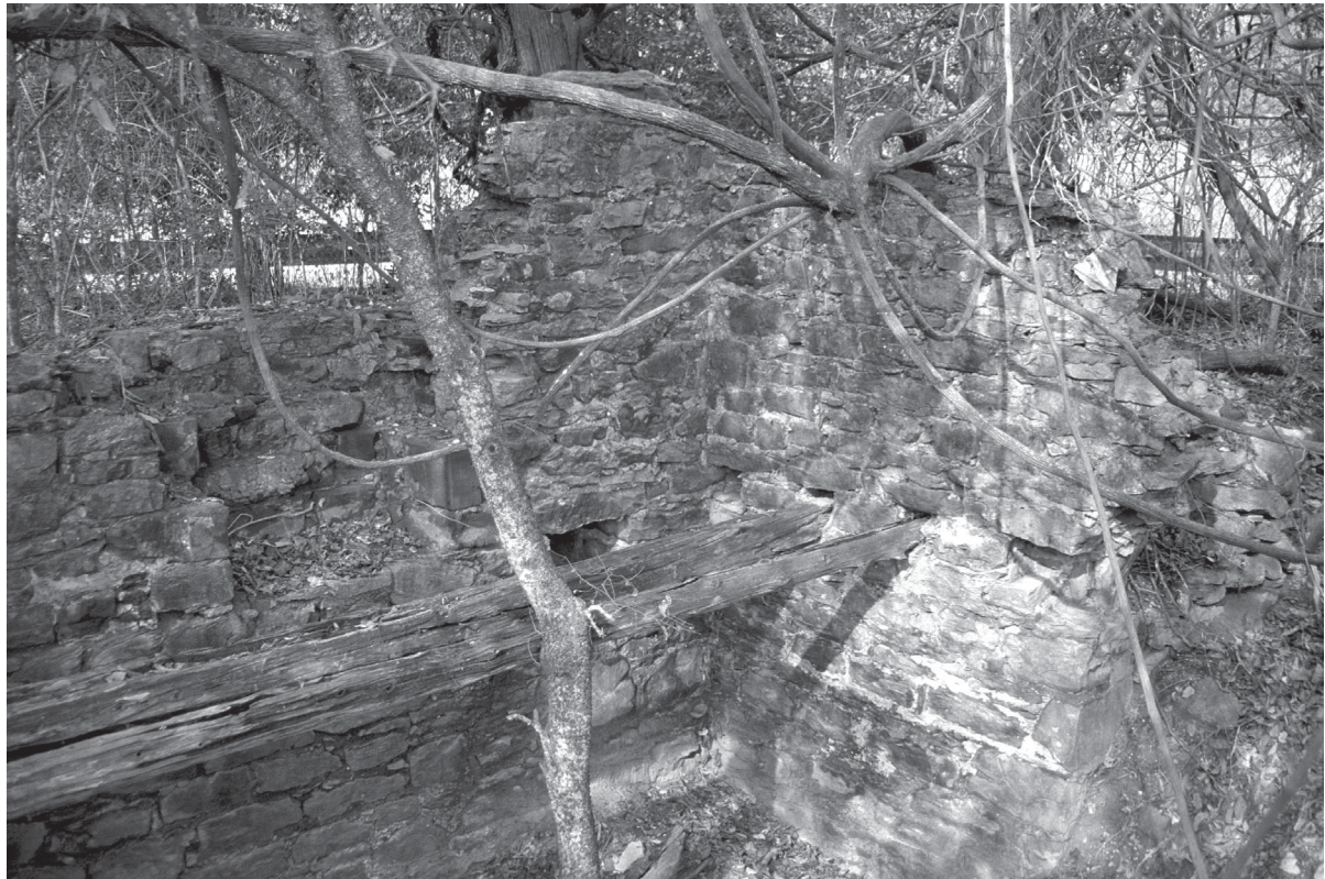
Figure 4-49. A few floor beams still remain; facing northwest.
