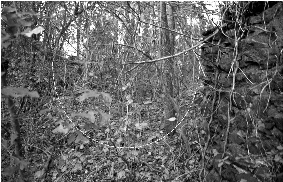
Figure 4-63. This photo shows the opening on west end of Aussiloux's dam, with the white line indicating where a metal conduit was installed to direct the flow of water into an irrigation ditch. The ditch ended nearly .7 mile at his grape fields.
