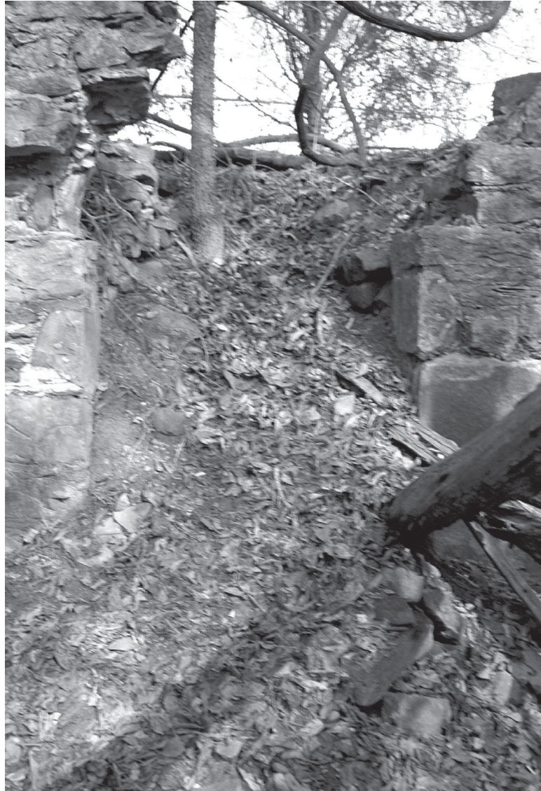
Figure 4-50. Debris-filled stone stairway leading from Aussilloux’s cellar; facing north.
