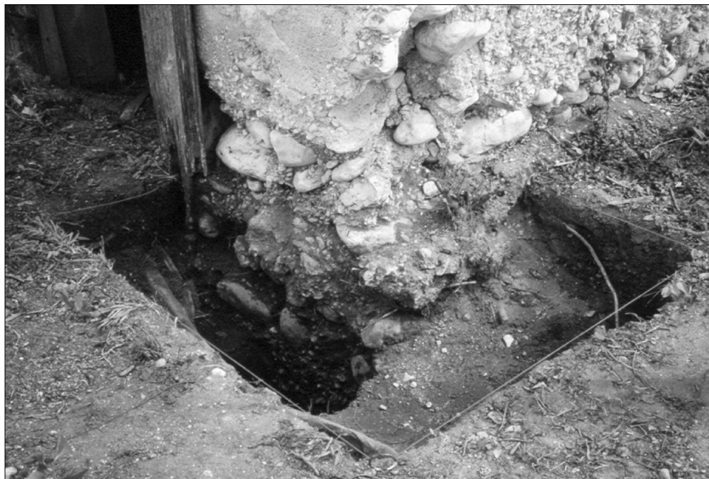
Figure 9. Base of wall and footing exposed in Unit 3 adjacent the southwest corner of the structure.
