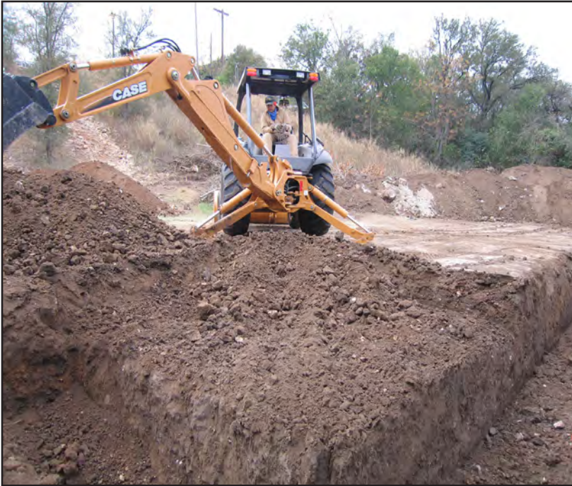
Figure 4.7. Mechanical stripping of overburden, facing southwest.
