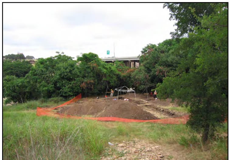
Figure 4.5. Overview of site after excavation of BHTs A and B, facing northeast.
