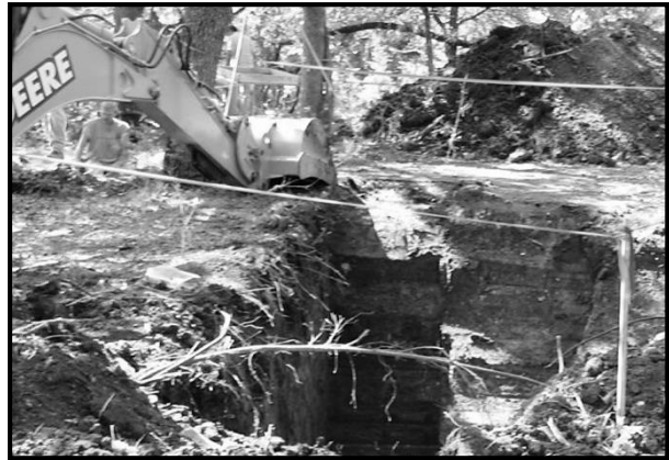
Figure 4-1. Example of trench excavation at sites.
