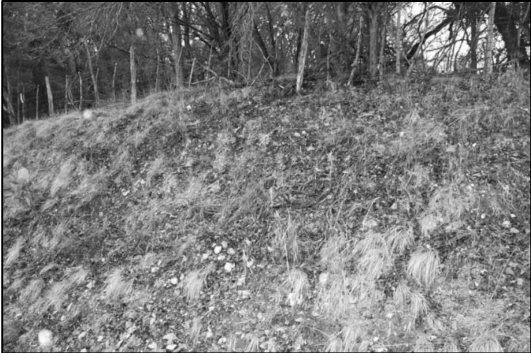
Figure 8-3. Eastern edge of existing right-of-way showing steeply sloping, eroding deposits of BRM 1 exposed beneath the existing fence at 41LM49 (photograph by Allen Bettis, May 2004).
