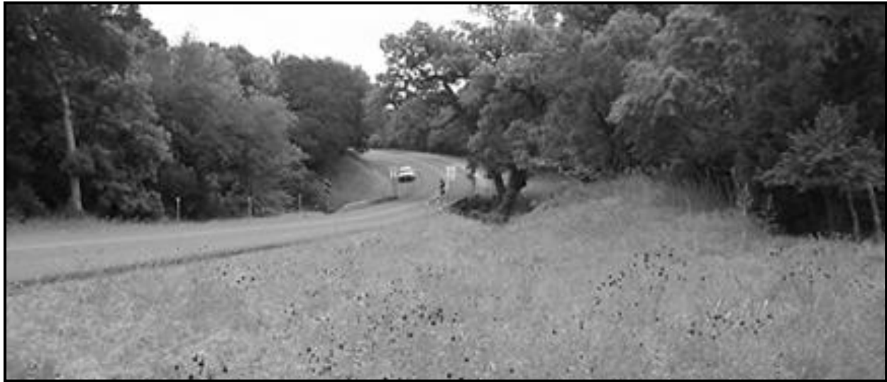
Figure 2-1. Overview of roadway crossing Lynch Creek (photograph by Allen Bettis).
