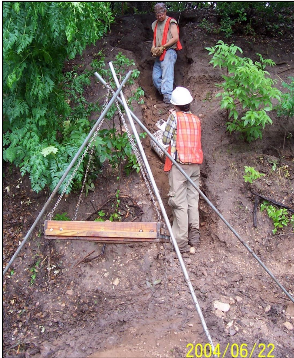
Figure 5-7. Example of excavation procedures on steep slope.
