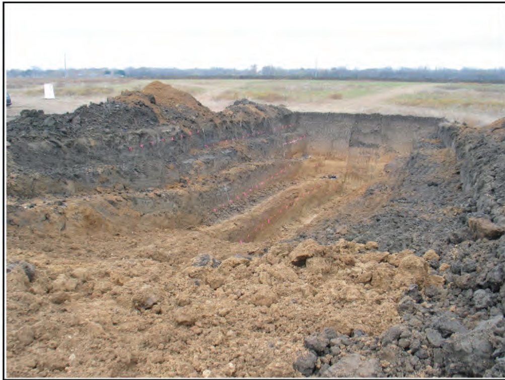
Figure 6-25. Photo of the deep trench in Area 2 as it appeared during profile drawing in December 2005.
