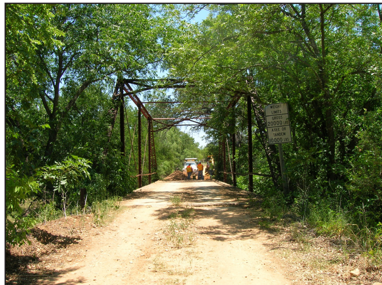
Figure 1.4. Existing bridge over Richland Springs Creek along CR 228.
