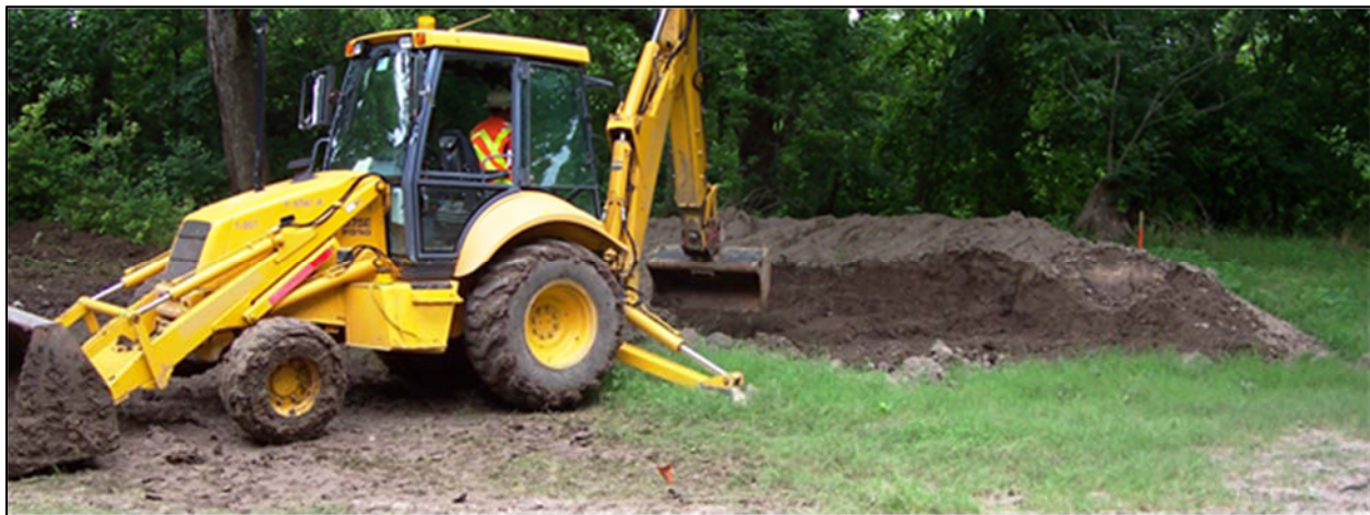
Figure 4-4. Backhoe removing sediments at Anomaly 3 at 41BL278.
