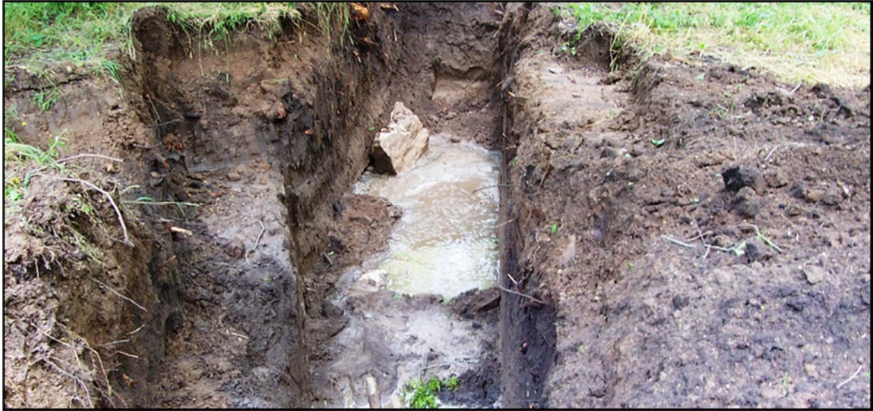
Figure 5-3. Backhoe Trench 12 with rain water and one of the two large rocks thought to represent Anomaly 3.
