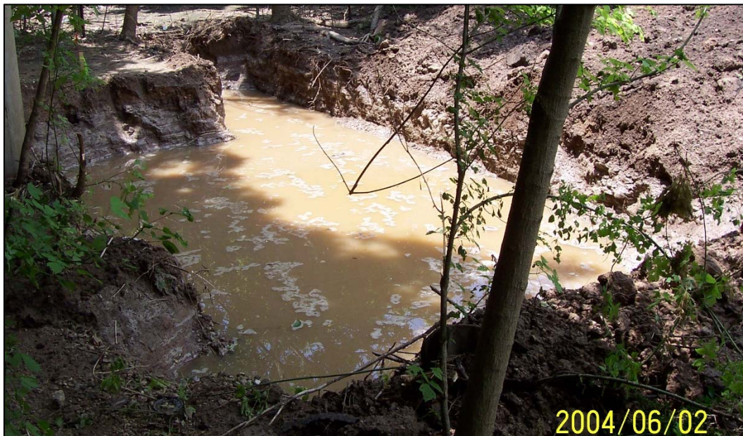
Figure 4-8. Backhoe Trench 11 and Test Unit 3 at Anomaly 1 filled with rainwater.
