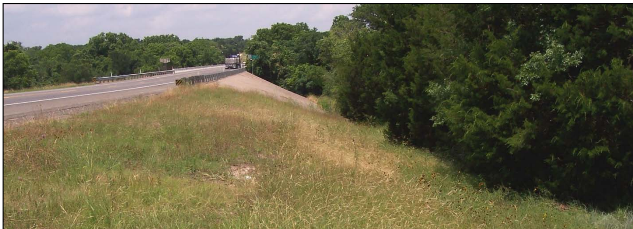
Figure 1-1. Overview of bridge location facing north.
