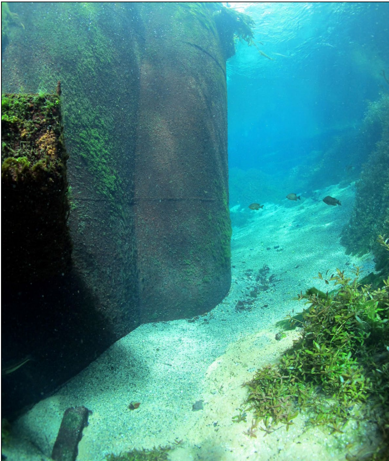
Figure 5-13. Rear of sub showing direct continuous contact between the lake bed and the base of the submerged structure.
