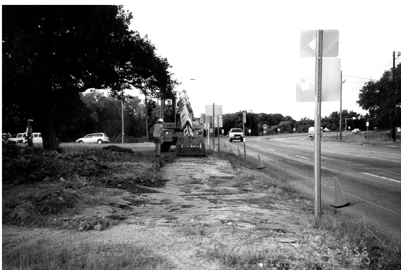
Figure 7-1. Area of investigations, 1998 –east side of US 77. Looking south.
