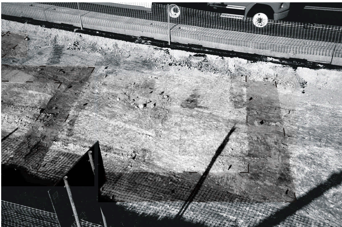
Figure 8b-7. Foundation trench of apse and south transept of Mission Refugio. Looking west.
