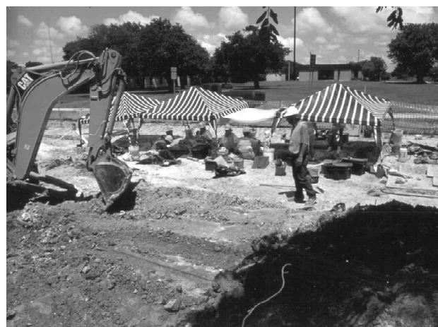
Figure 7-4. Archaeological monitoring of Gradall excavations at Mission Refugio.
