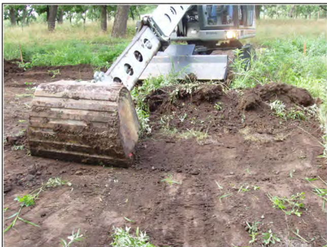
Figure 4-8. The Gradall bucket was floated in order to grade in 10-cm intervals.
