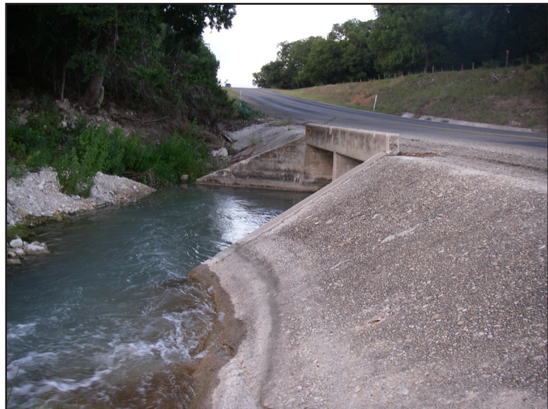
Figure 1.3. Existing box culverts under FM 2169 at Johnson Fork (facing south).
