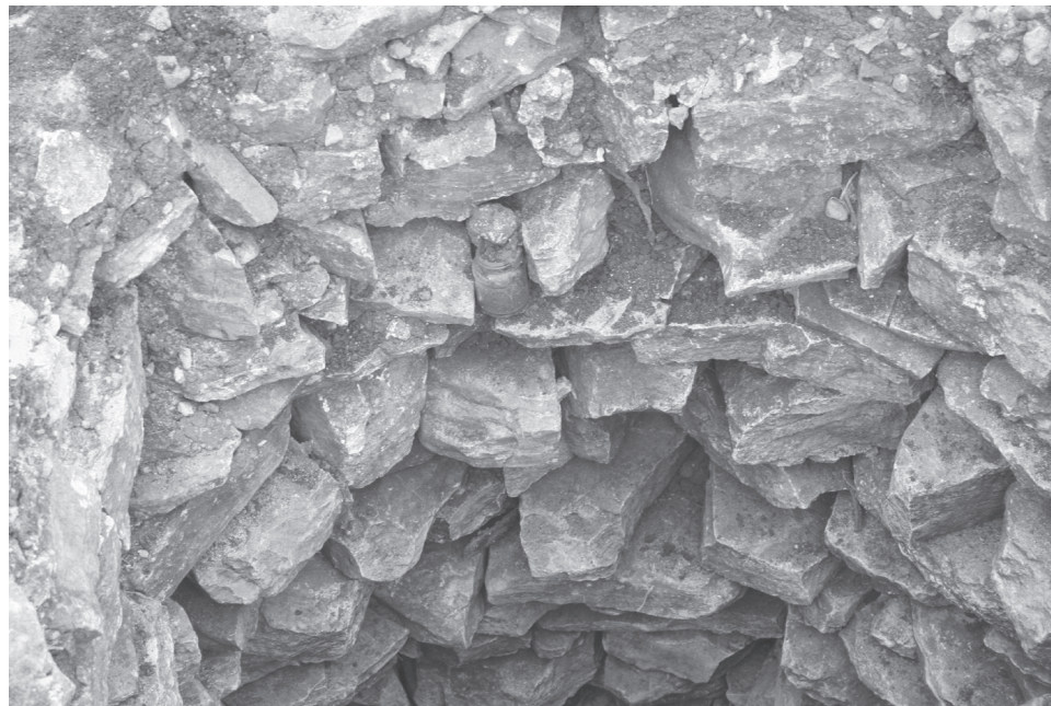
Figure 5. Close up of well wall illustrating dry stack construction technique.
