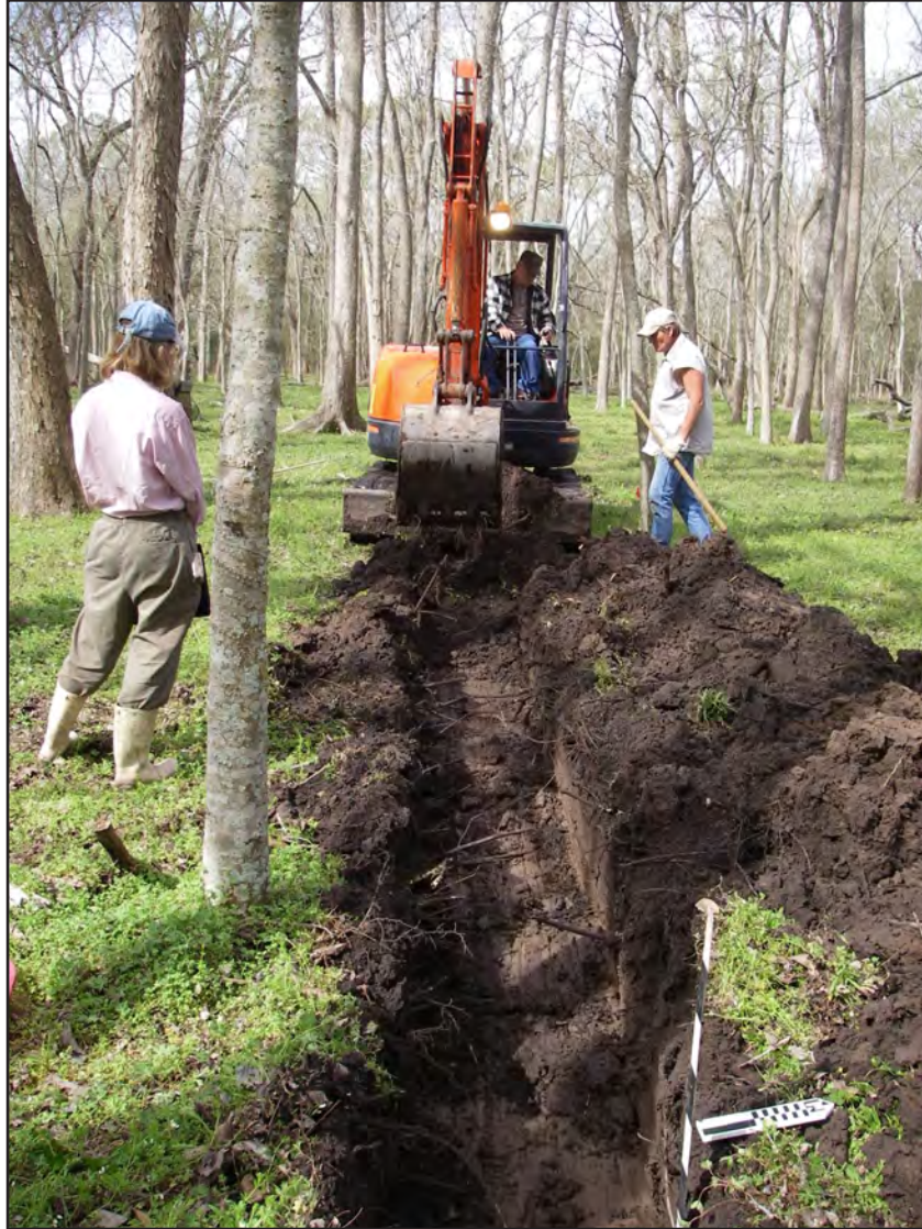
Figure 9-3. Monitoring of mechanical stripping at site 41CH371. View is to the west. Date: 3/2/07.
