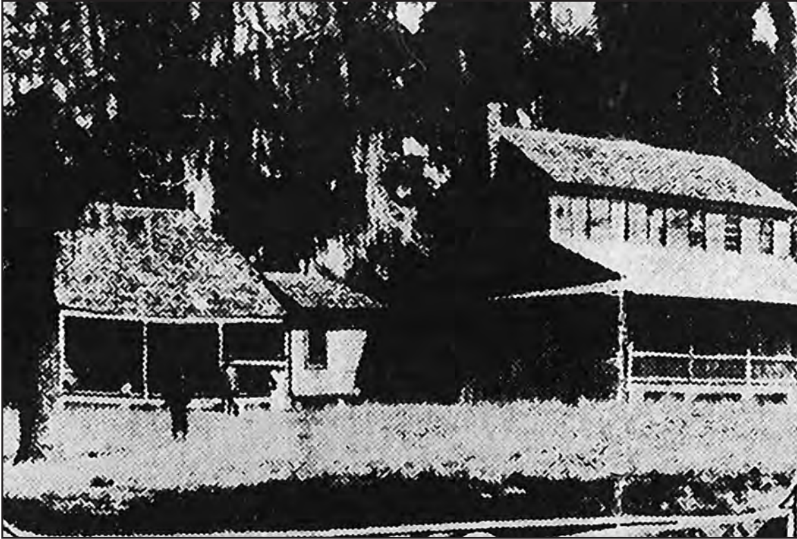
Figure 4-1. Taylor White's first home was most likely the building on the left. Historic documents suggest that White built the larger, second home (on the right) sometime later. View to the northeast. (After Sunday Enterprise 1935, JVCC.)
