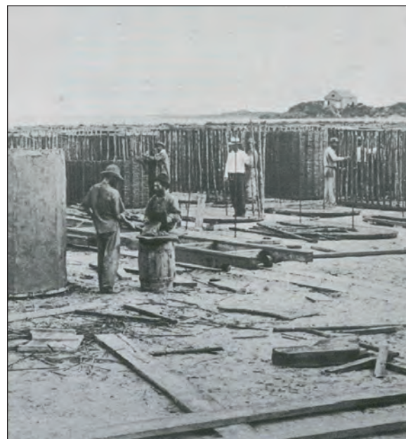
Figure 3. Gabion construction at Point Bolivar (source Alperin 1977).
