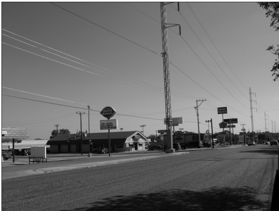
Figure 2. Between Ingram and Oak Knoll, Callaghan Road is commercially developed and retains little potential for encountering intact cultural or buried deposits.
