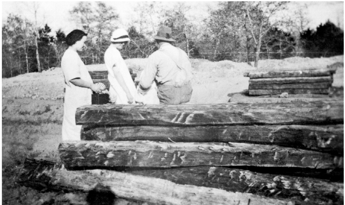
Figure 3. Railroad ties for the spur being built from the Sayers Mine to the MKT line, ca. 1914. From left to right: Sue Smith, Mrs. J. D. Owens, and J. D. Owens, the supervisor of the mine. (Photograph in the Camp Swift historical files, AGTX-EV, Camp Mabry.)
