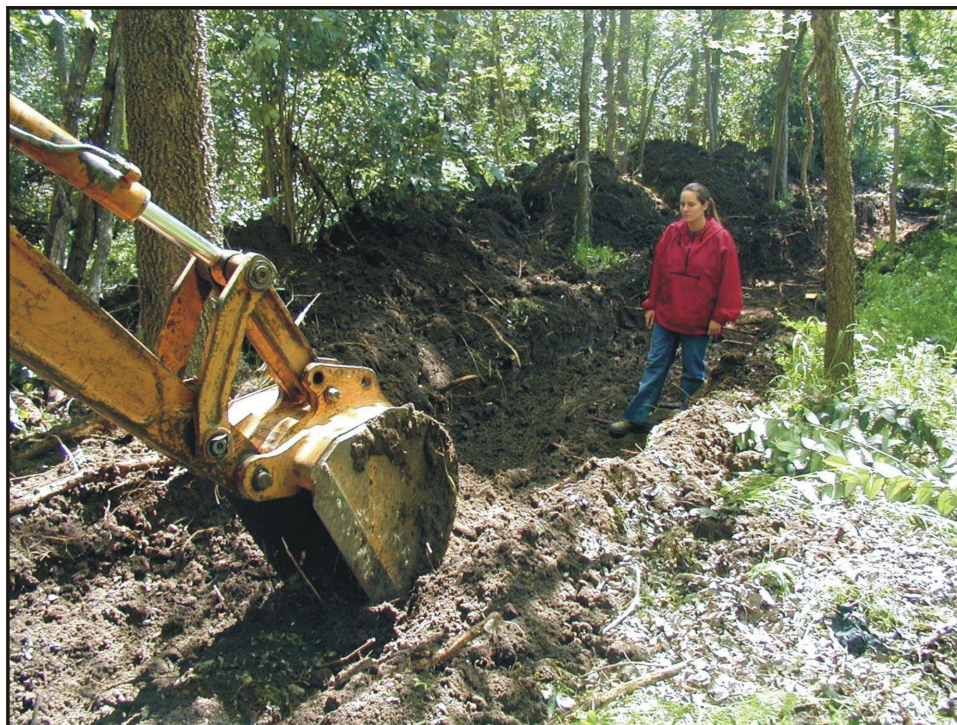
Figure 12. The excavation of Backhoe Trench 7.
