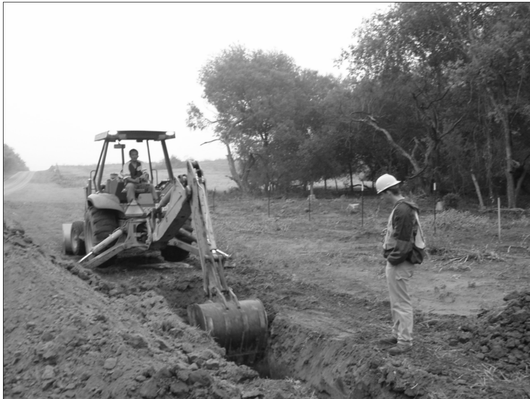
Figure 3-2. Backhoe trenching at FM 536.
