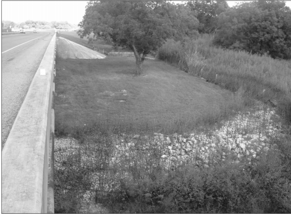
Figure 1-3. Photo overlooking Area 1.
