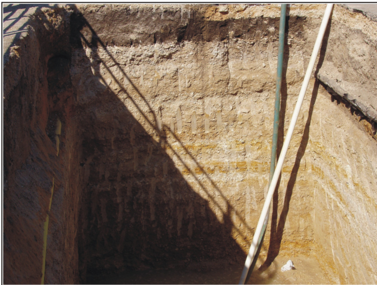
Figure 4-15. Deep pit dug in E. White Avenue west of Mission Road at the time archaeologists arrived at the site.
