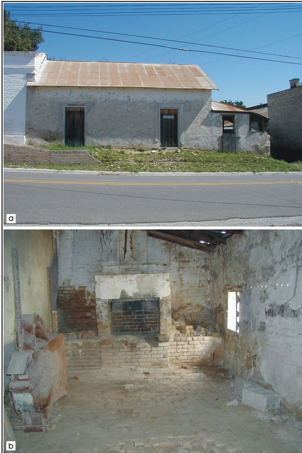
Figure 2-4. The Stone Cottage (41SR211), February 2003. (a) front of cottage facing Portscheller Street; (b) interior of the addition with kitchen fireplace.
