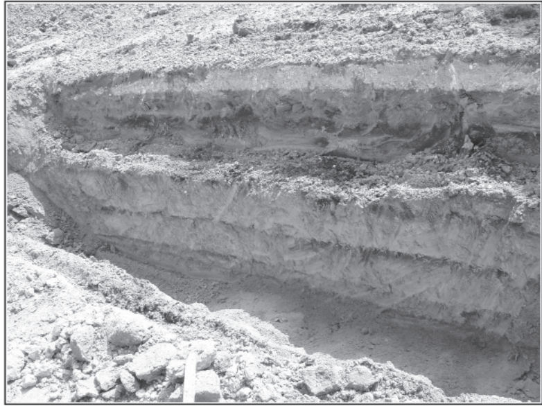
Figure 4-1. Trench with sides stepped down to allow CAR monitors to enter safely.
