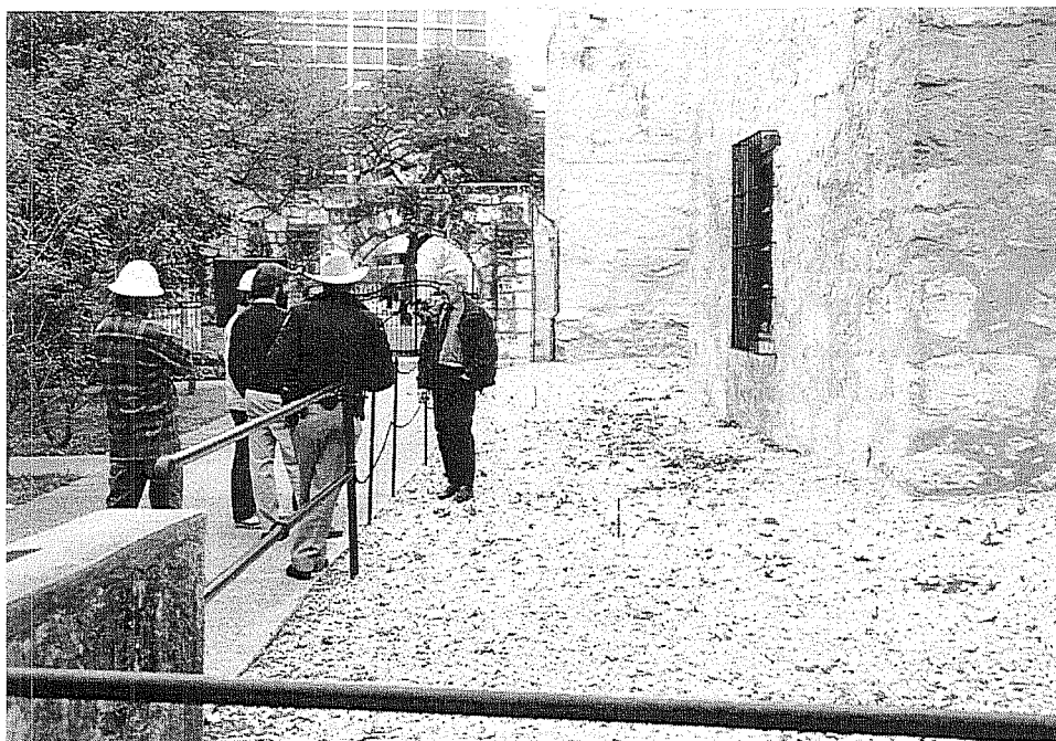
Figure 16. Area of exterior excavation, before project, looking west.
