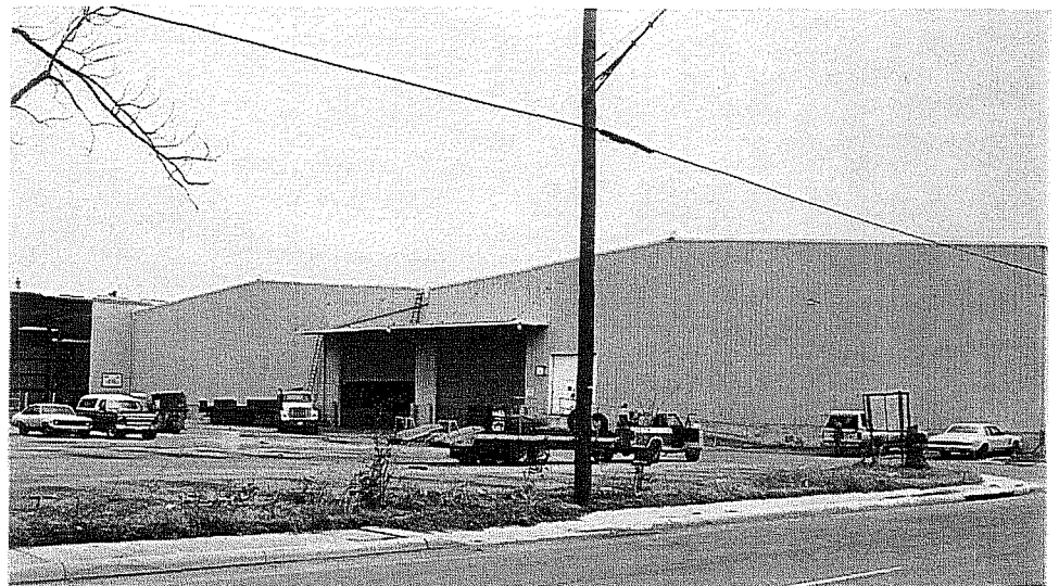
Figure 3-12. Main Warehouse and Re-bar Fabrication Shop, north facade.
