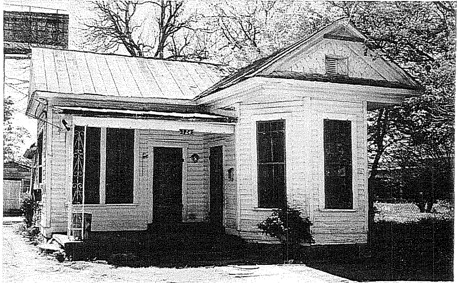
Figure 3-19. Plains cottage . 124 Nevada Street. APA 1990.
