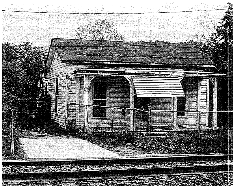
Figure 3-18. Hall and parlor house. 106 Martin Luther King Street. APA 1990
