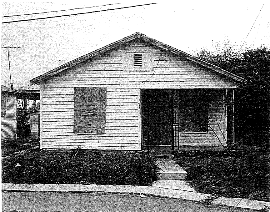
Figure 5-1. Small frame bungalow at 123 Runge Street, 1990.
