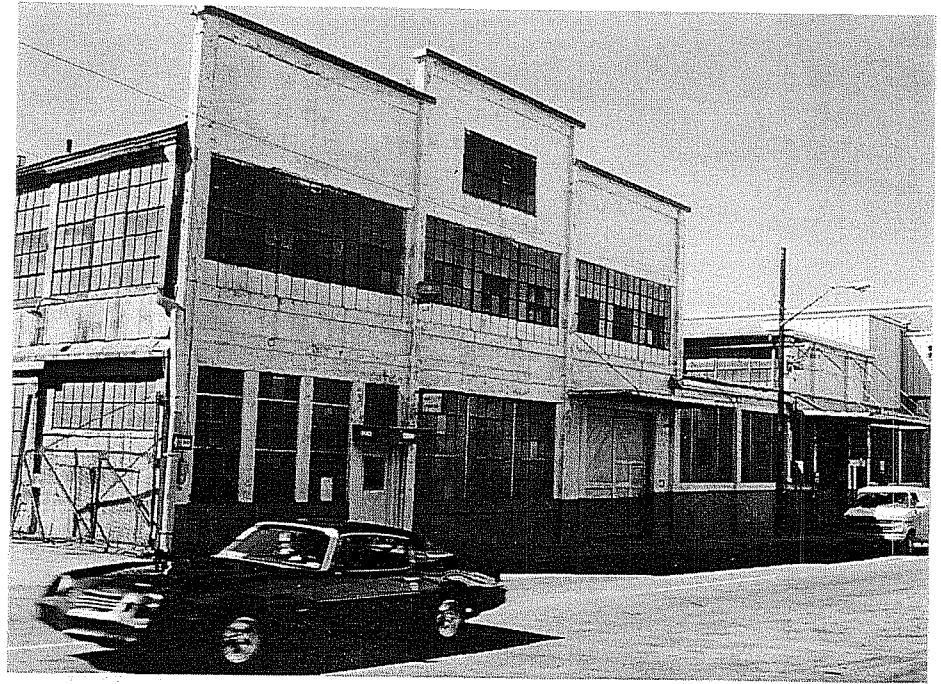
Figure 3-9. Alamo Iron Works, the oldest existing shops.
