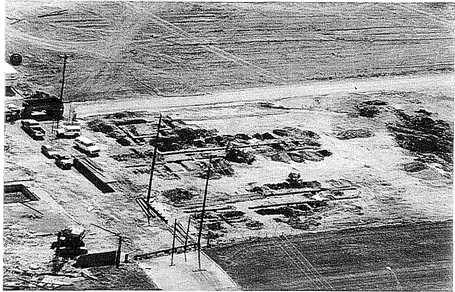
Figure 4-29. NCB 613, north excavations. Facing southeast.
