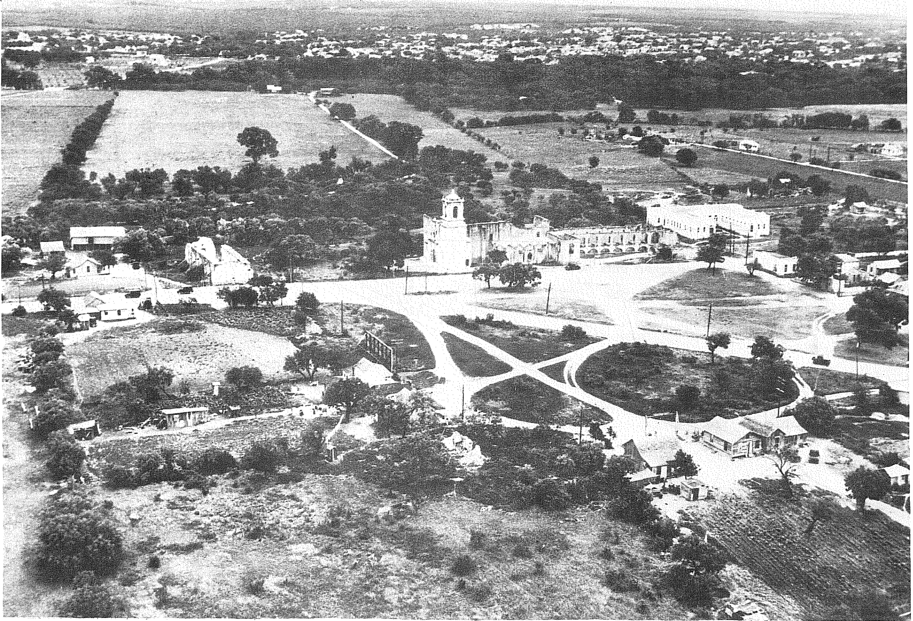
Figure 3. Undated Aerial Photograph of Mission San José Looking North-Northeast ca. 1931-1932. From the files of the San Antonio Missions National Historic Park. Note Schelcher property outlined by trees in lower left quadrant, and privy near the north lot line. For location of backhoe trench, compare with Figure 2.
