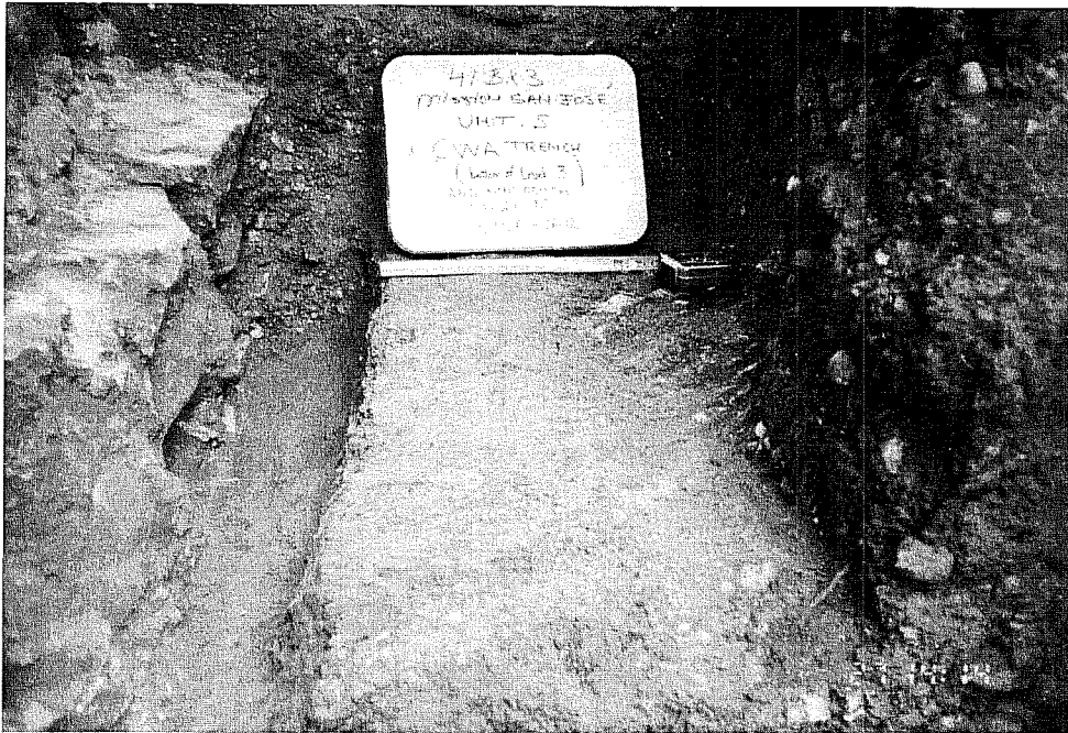
Figure 4. Outline of the exterior CWA trench. Note depth and width away from wall base.
