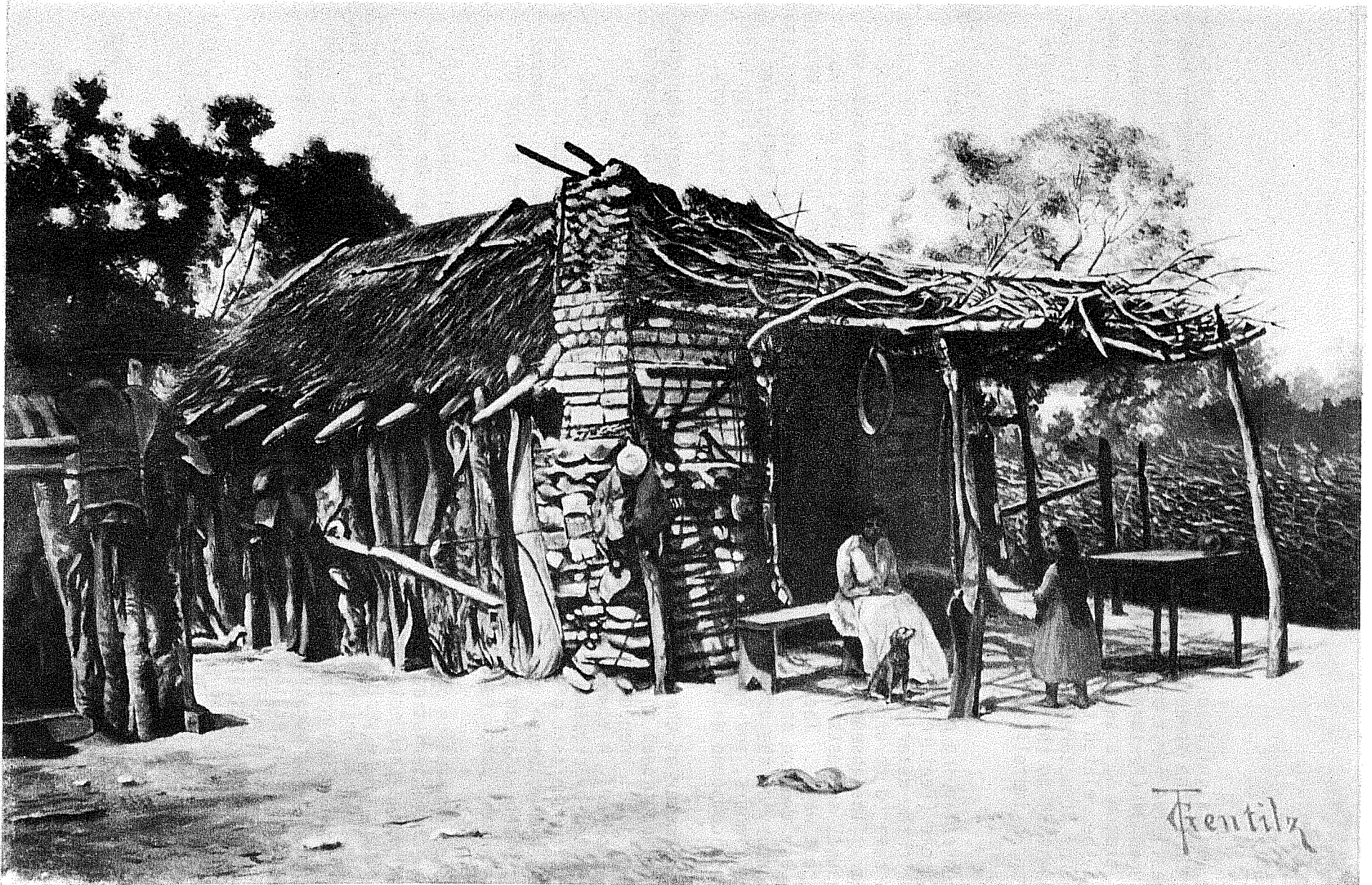
Figure 11. Jacal in San Antonio, Mid-19th Century. This painting by artist Theodore Gentilz shows the typical jacal made of upright poles and thatched roof. The structures within the compound at Rancho de las Cabras probably looked very much the same.
