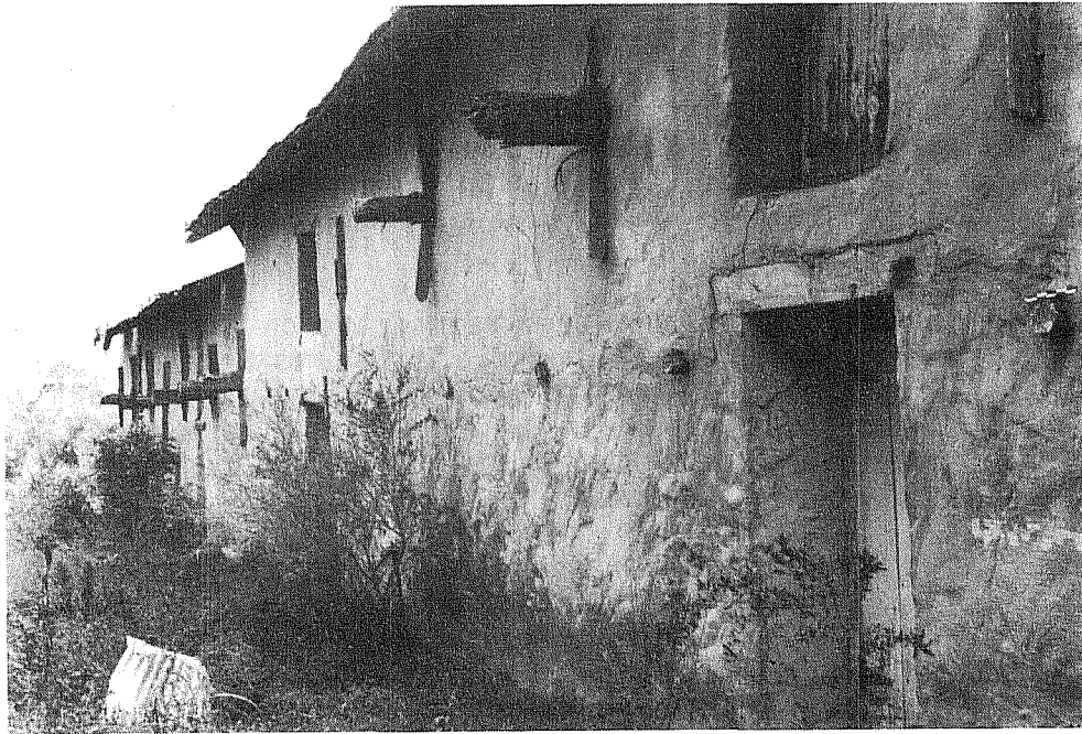
Figure 39. Barn Structure at 41 BX 664. View towards the east.
