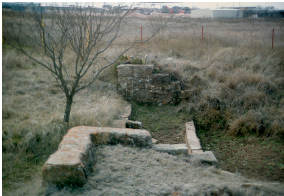
Figure 4. Check dams at site 41BR270. Photos by Alan Wormser, 1994.
