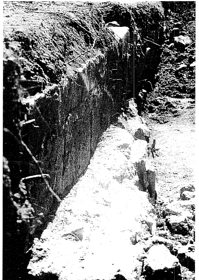
Figure 7. Upper Labor dam stonework. Nineteenth century ashlar-dressed limestone (upper), undressed Spanish colonial limestone (bottom).
