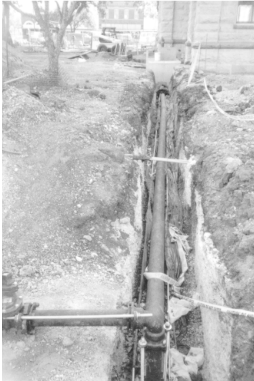
Figure 2. Fire line trench on NW side of courthouse lot.
