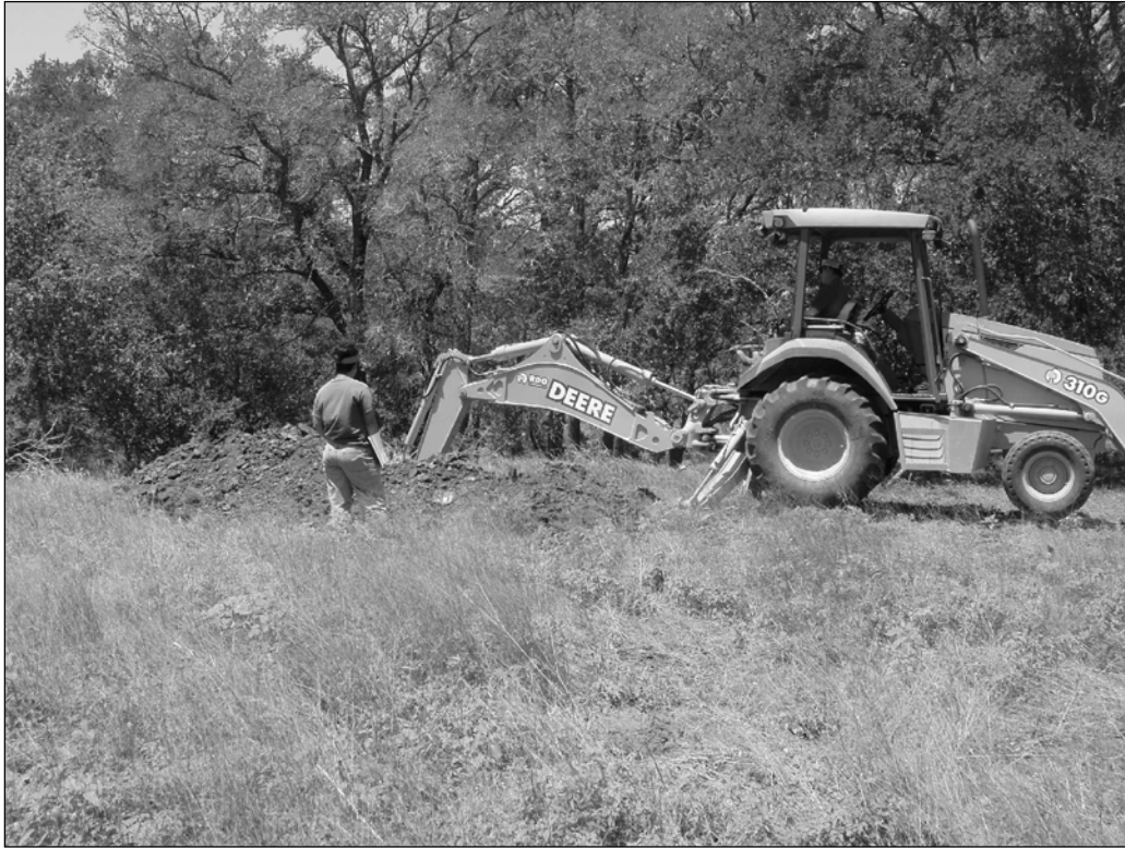
Figure 5-2. Backhoe trench excavation at 41BP679.
