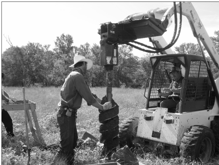
Figure 5-1. Mechanical auger in use on site.
