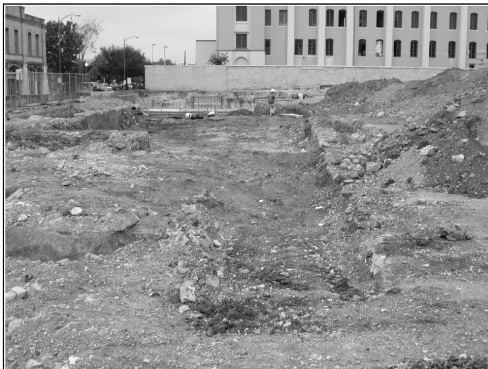
Figure 5-9. Photograph of the initial bladed area, looking north.
