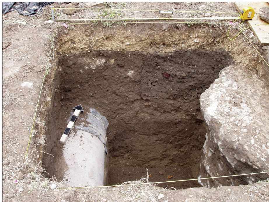
Figure 3-11. Pipe and buttress exposed in Unit F.
