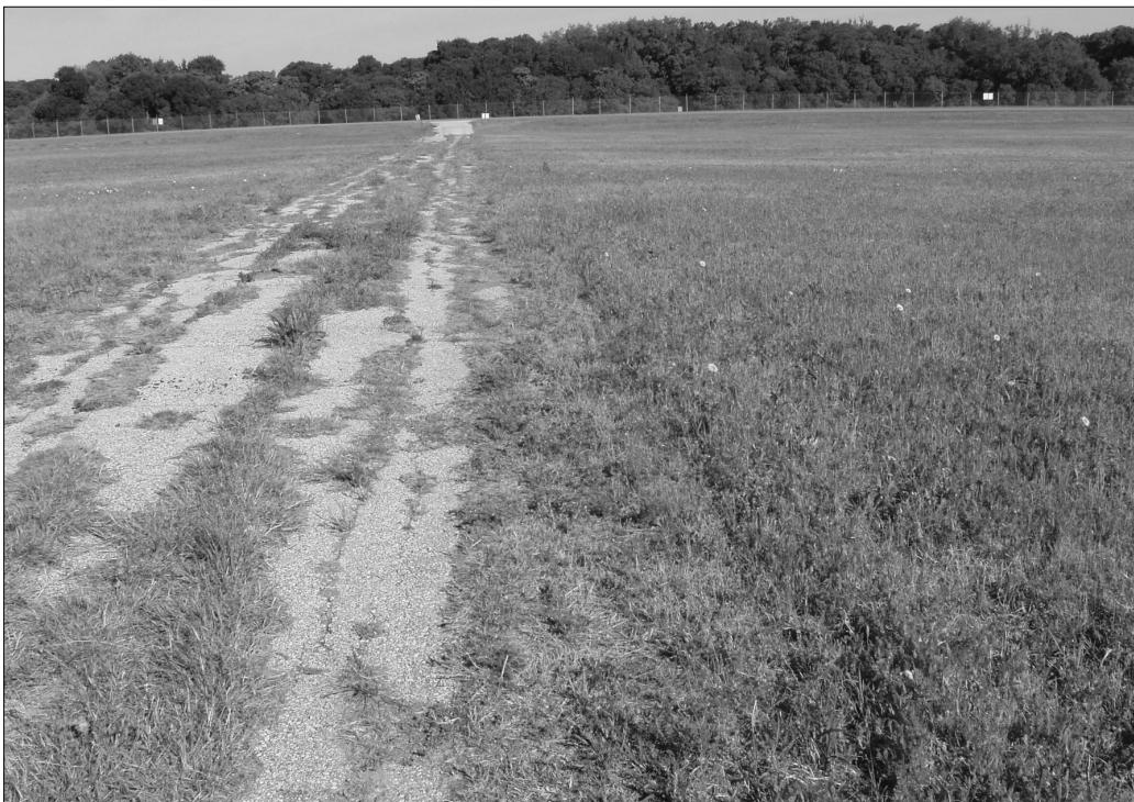
Figure 4-10. Paved roadway that crosses the southern portion of Tract 2.
