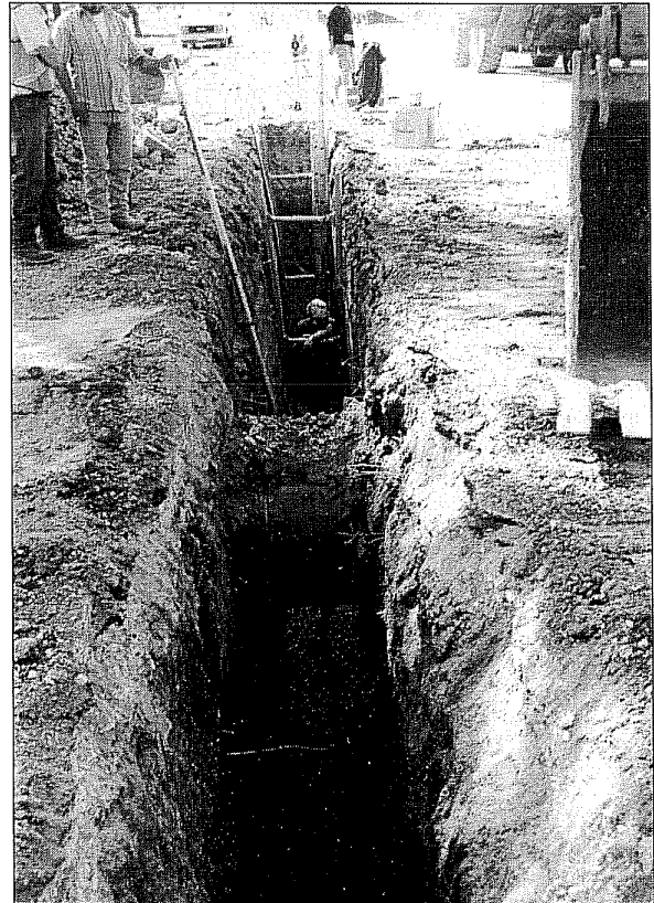
Figure 5-7. Photo showing trench for Drainage System A storm sewer passing under reinforced concrete pipe carrying the Espada Acequia.
