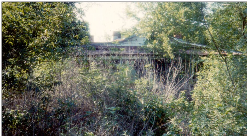
Figure 4-8. 1950s structure on site 41BX347.
