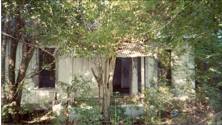
Figure 4-7. 1940s structure on site 41BX347.
