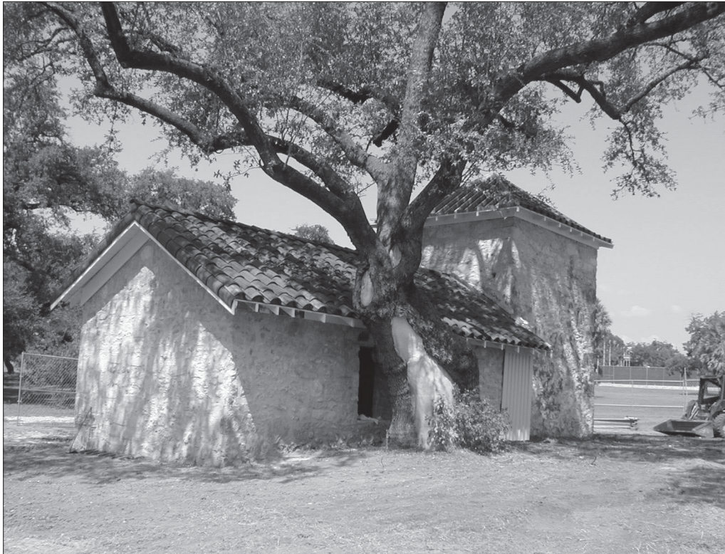
Figure 2. The Block House in 2002, during renovation.
