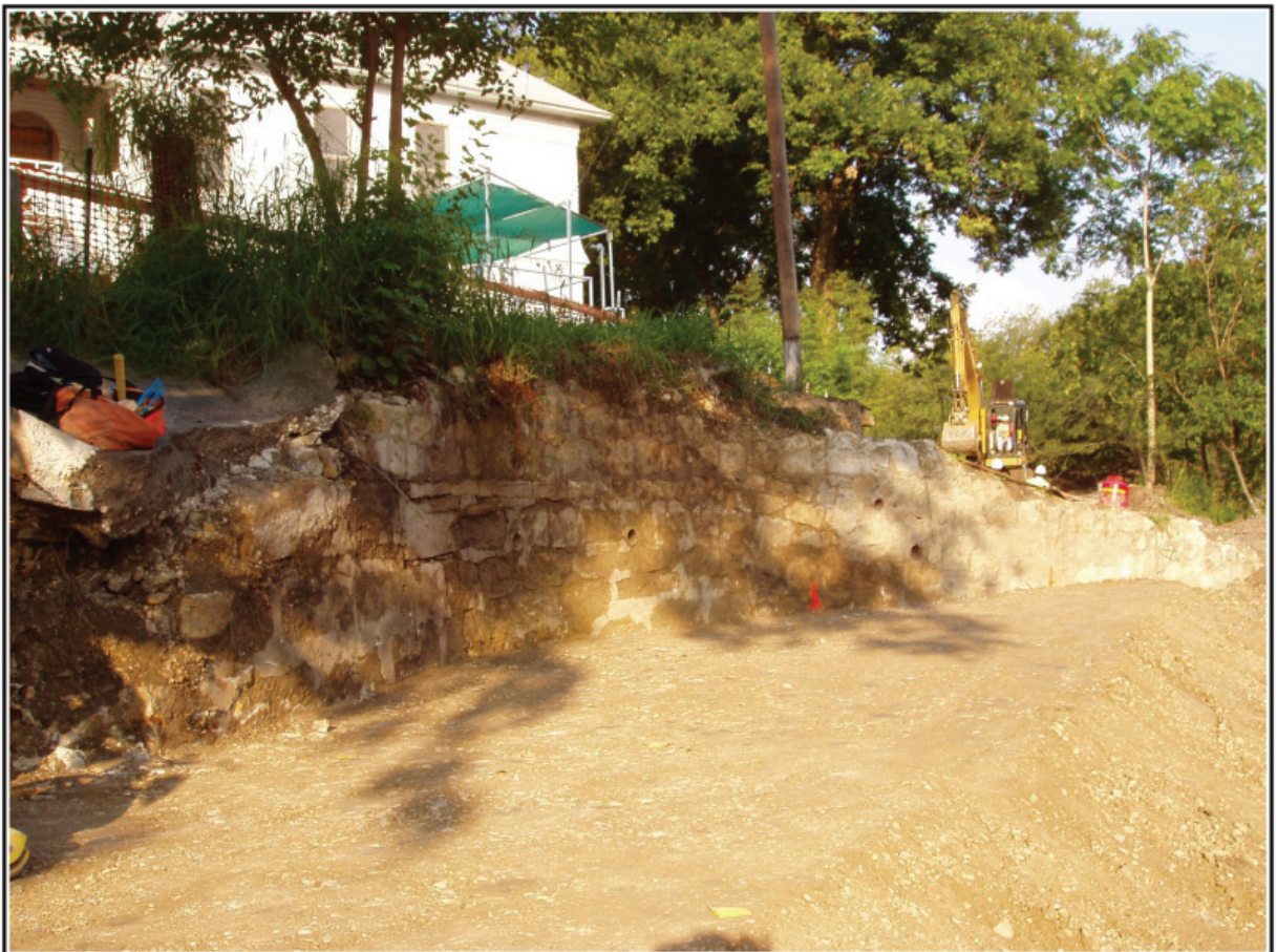
Figure 4-23. Feature 10, the stone wall located near the VFW Post #76 (see Figure 4-1).
