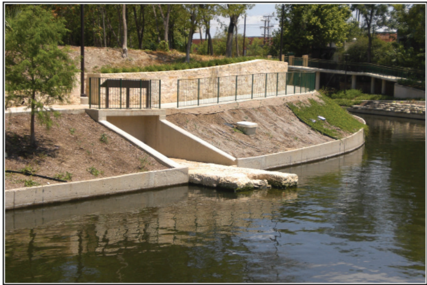
Figure 6-1. The Alamo Mills Dam as it is seen today.
