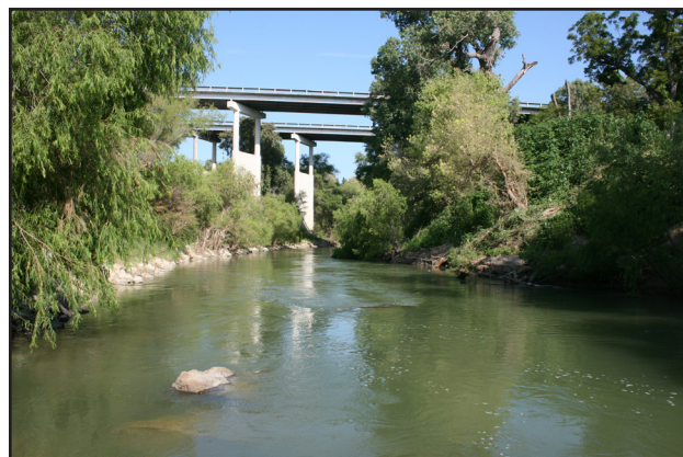
Figure 2.1. San Antonio River flowing southeast beneath the IH 37 bridge.
