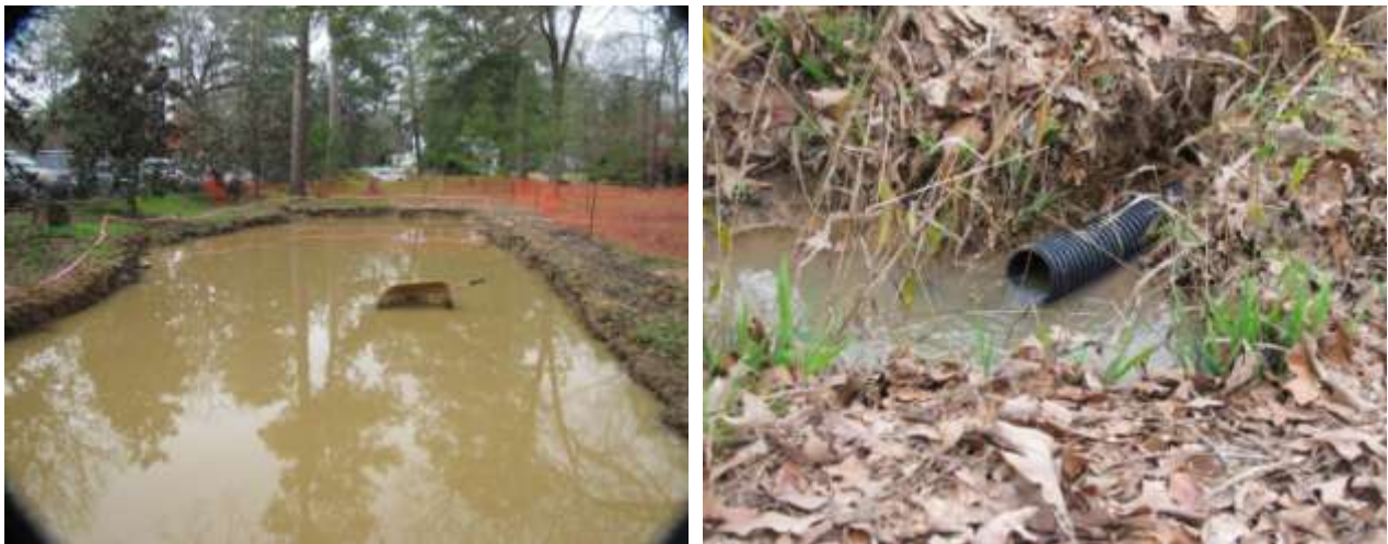
Figure 4. Rain Gardens work! Muddy water goes in, clear water comes out. Photos by Yanli Zhang.
