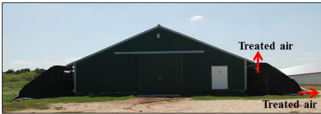
Figure 4. Biocurtain covering the entire exhaust area on both sides of the treatment house. Treated air leaves vertically and through the opening near the bottom corner of the structure.
