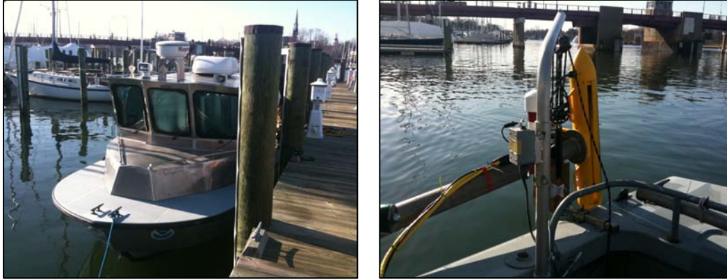
Figure 10. Teledyne Benthos C3D installation on NOAA R/V Lookdown.
