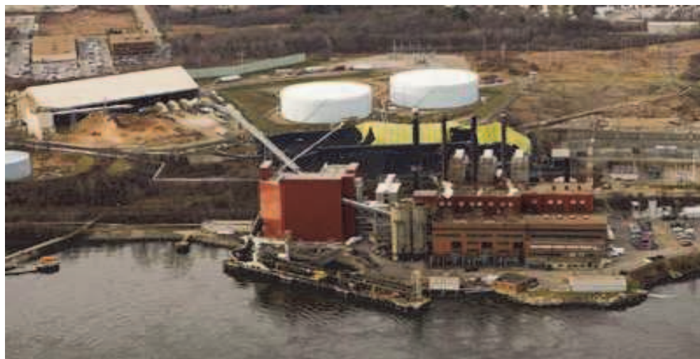
Fig. 5. Schiller Station, Portsmouth, NH.
