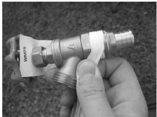
Step 4: Wrap silicon tape around threading on spigot 2-3 times
