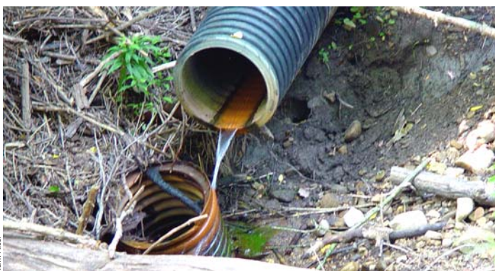
Pipe discharging water during dry weather
